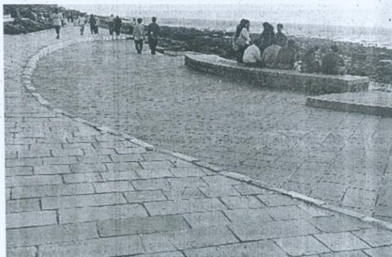
Bandra Bandstand after the redevelopment work
