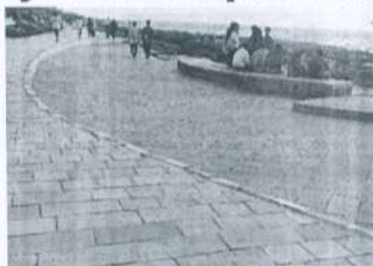
Bandra Bandstand after the redevelopment work
