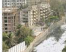
RIVER OF MUMBAI Storm and garbage problems on the banks of the River Worli, while on the opposite bank, greenery has been restored. The right is view from an area just above the river where the nullah was constructed and left to drain and pollute in the monsoon days.
