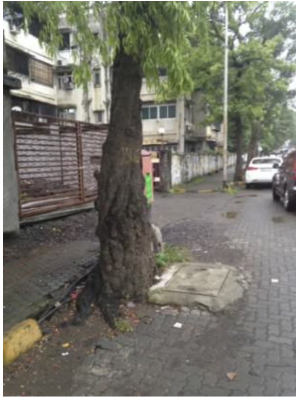
A drain and its chamber has to be right under the trees? Photo: P.K. Das
